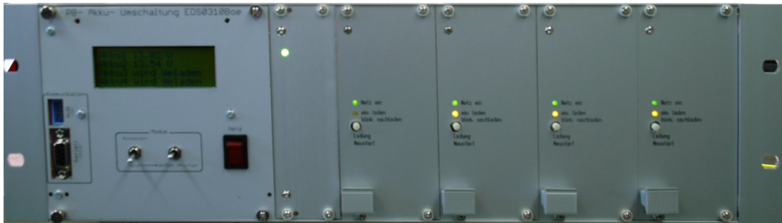
Figure 2.18.: Low noise battery power supply: In the left part the display and control unit and in the right part four separate charging circuits, each connected to one battery
